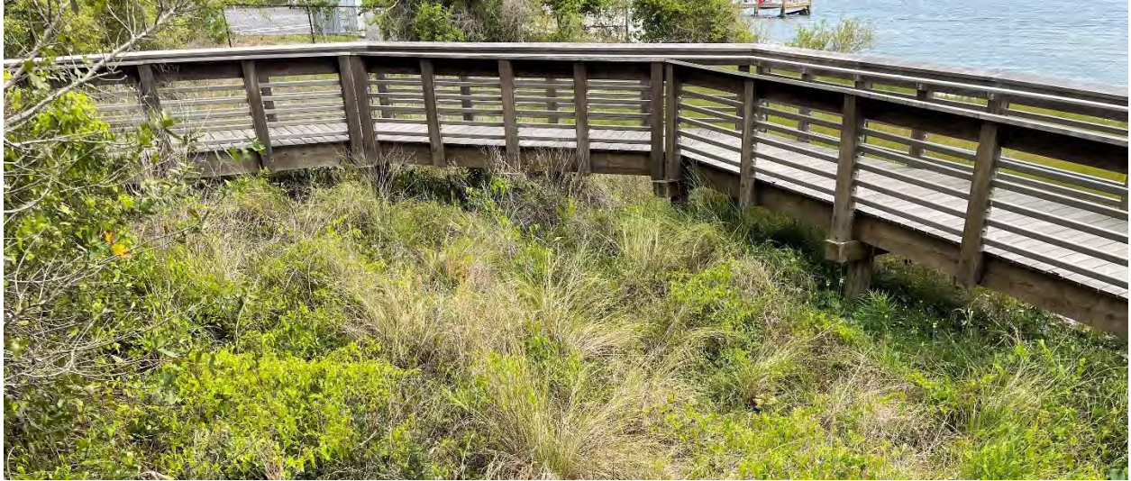
View of the access boardwalk (looking southeast)
