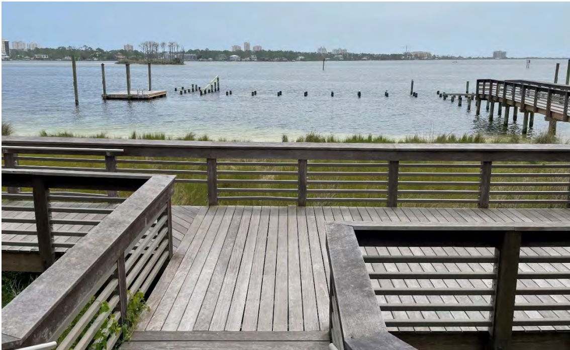
View of the access boardwalk (looking south)
