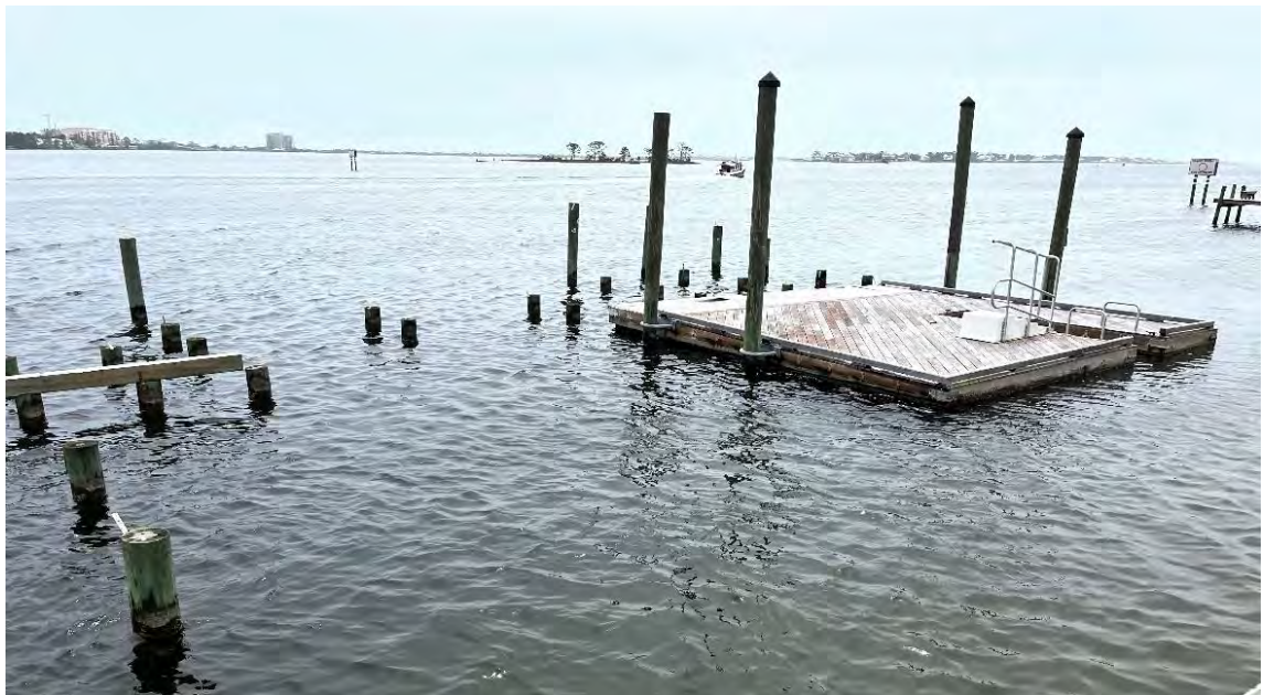
View of remaining dock piles and paddle craft access (looking southwest)
