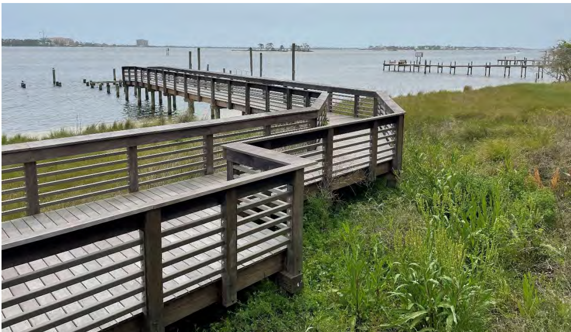
View of the access boardwalk and remaining dock (looking southwest)
