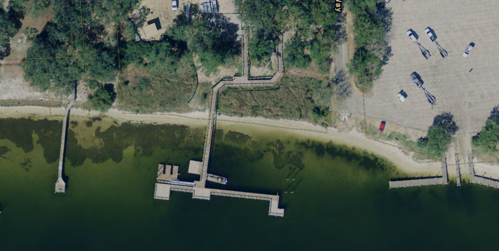
FDEP Map Direct Image (unknown date) - Dock is under construction
