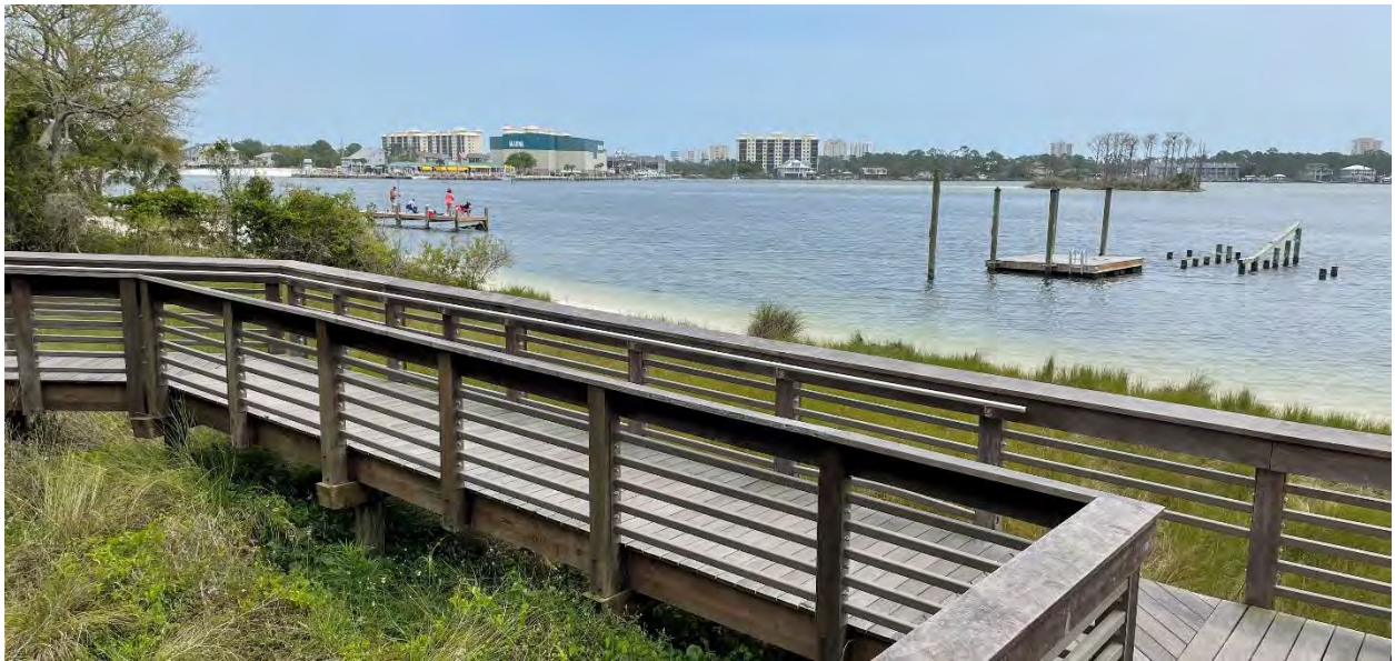
View of the access boardwalk (looking south/southeast)
