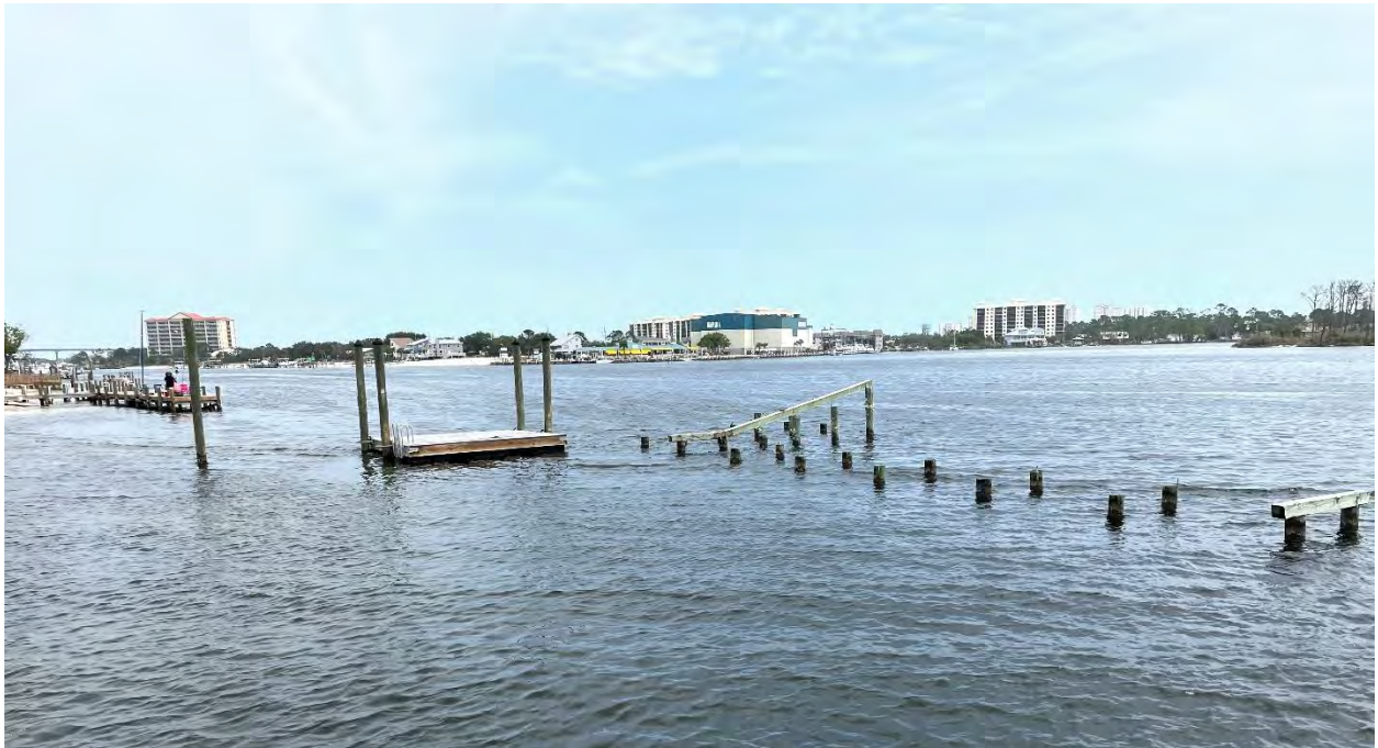
View of swimming pier and remaining dock piles (looking southeast)
