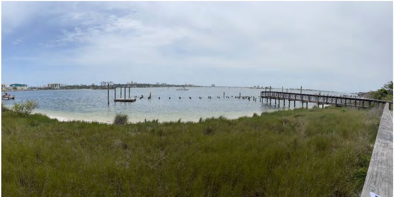
View of swimming pier, remaining dock piles, and remaining dock (looking southwest)
